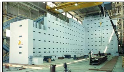
RTMD Equipment Site
